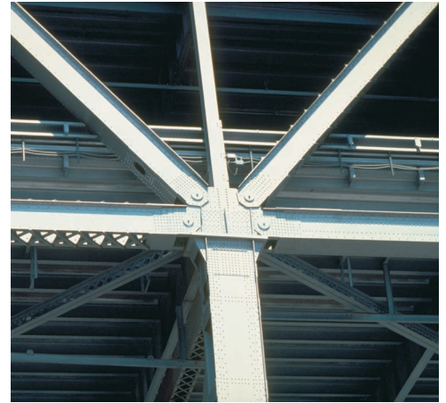
Photo 6.1 Shown is a pin-jointed connection on the approach span to the San Francisco–Oakland Bay Bridge.
