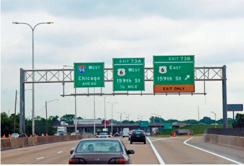
Photo 3.4 The parallel wind forces acting on the highway signs can be reduced to a single equivalent force. Determining this force can simplify the calculation of the forces acting on the supports of the frame to which the signs are attached.
