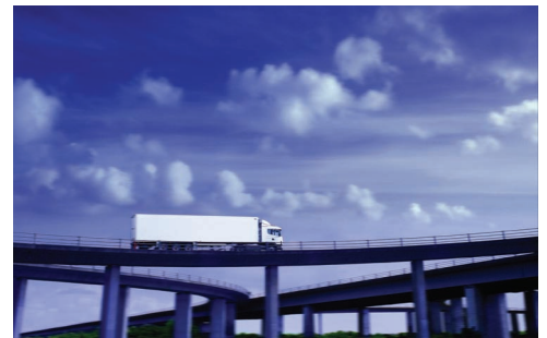
Photo 7.2 The internal forces in the beams of the overpass shown vary as the truck crosses the overpass.
