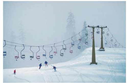
Photo 7.3 Since the weight of the cable of the chairlift shown is negligible compared to the weights of the chairs and skiers, the methods of this section can be used to determine the force at any point in the cable.
