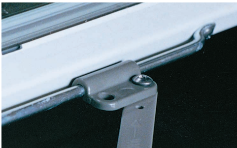
Photo 4.3 As the link of the awning window opening mechanism is extended, the force it exerts on the slider results in a normal force being applied to the rod, which causes the window to open.
