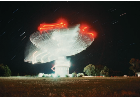
Photo 18.3 The revolving radio telescope is an example of a structure constrained to rotate about a fixed point.
